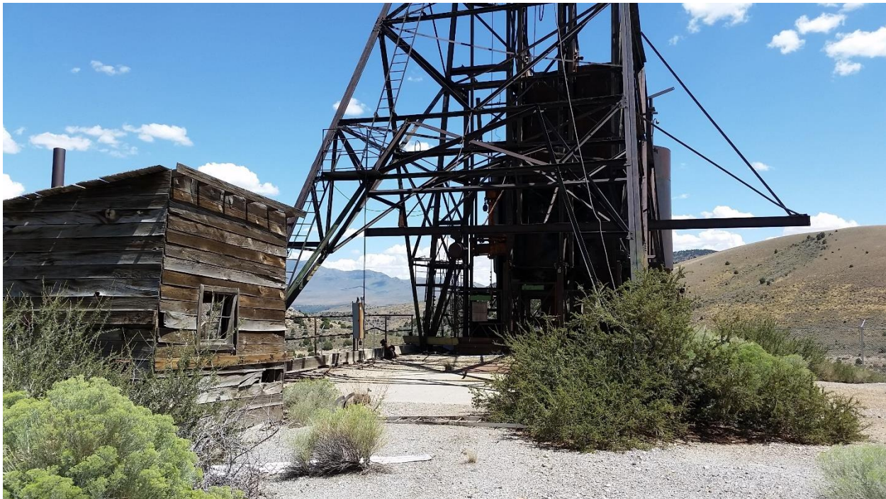
Photo 4-1: FAD Shaft Headframe and Hoist Building
