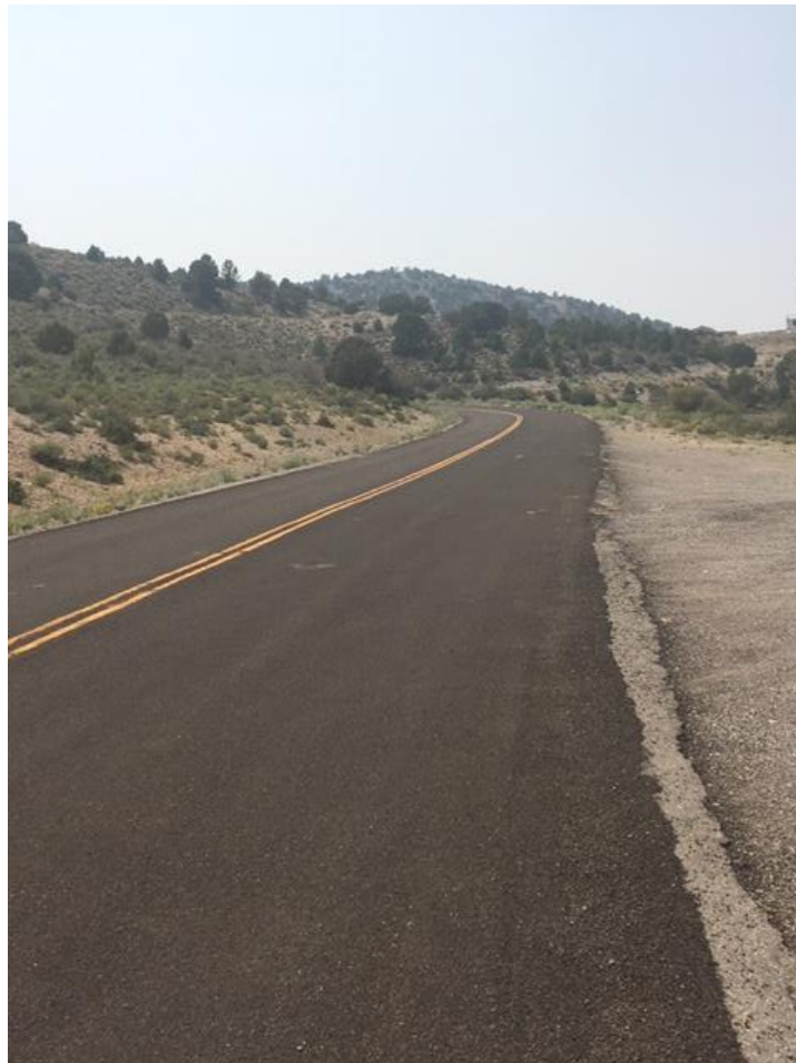
Photo 12-1: Asphalt Access Road from Eureka to the FAD Property
